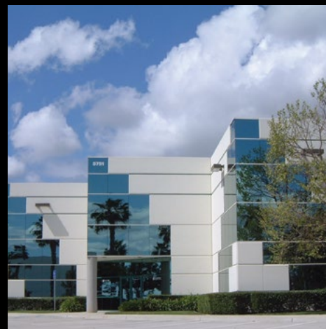
TELECOM BUSINESS CENTER
