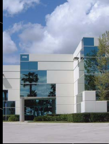
Telecom Business Center
