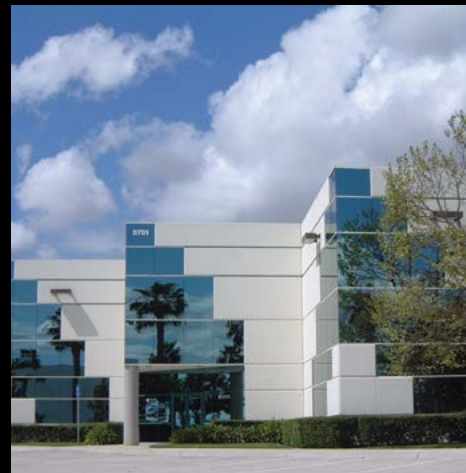
TELECOM BUSINESS CENTER
